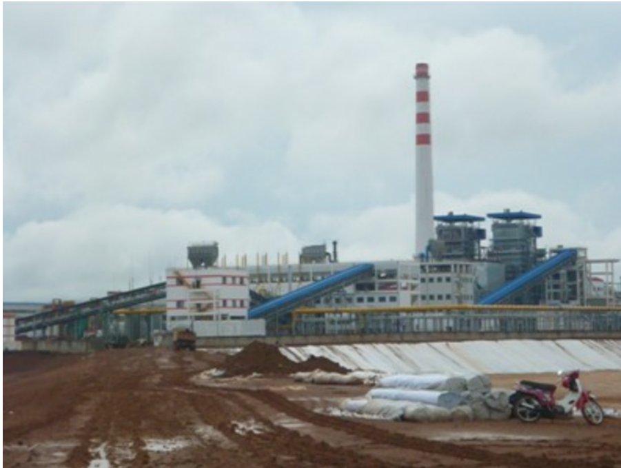
Figure 4. Tan Rai alumina plant, Vietnam.
